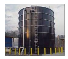
With existing certification for potable water storage for ISOFUSION® and TRIFUSION® to NSF/ANSI/CAN 61 and approval by the UK Secretary of State under Regulation 31 for drinking water and listed by Drinking Water Inspectorate (DWI) in its List of Approved Products, PERMASTORE® tanks are proven to be ideal for process water applications.
